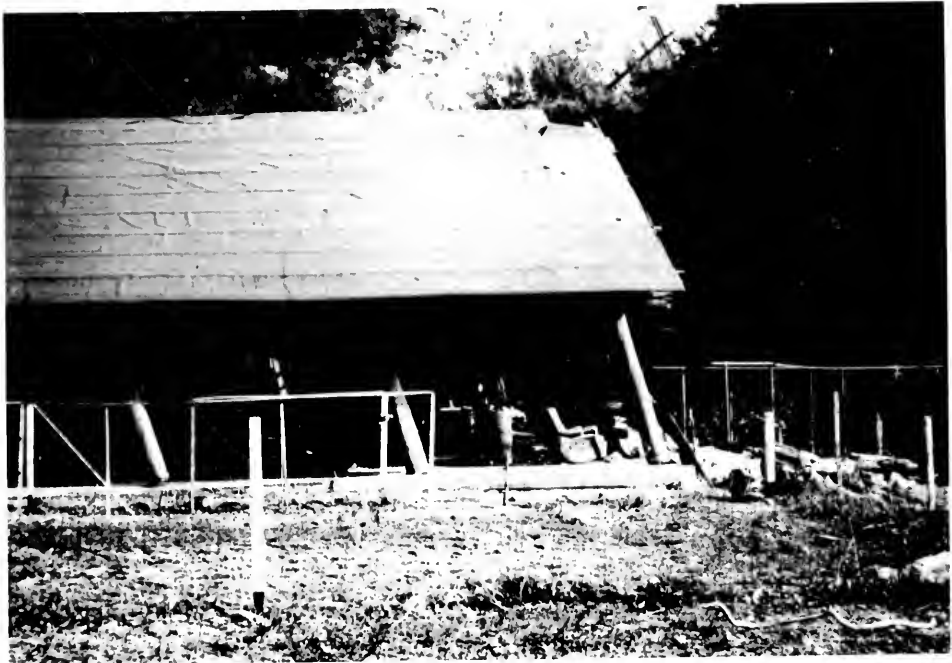
Photo 19. View east at a log lodge north of Wilson Canyon flood control dam and 670 m (2200 feet) north of the main building at Olive View Hospital. The inertial effect of severe ground motion on the roof has offset the roof N. 24° E.
